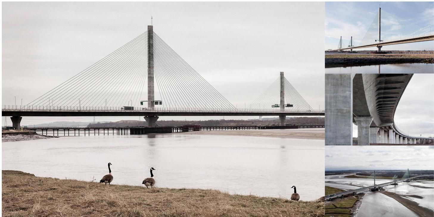
Mersey's bridge is a continuous structure 2248 m long without intermediate expansion joints. The central part (around 1000 m) is a four spans cable stayed structure.
